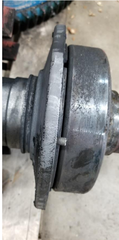
Broken Bolts on DE Bearing Cap
